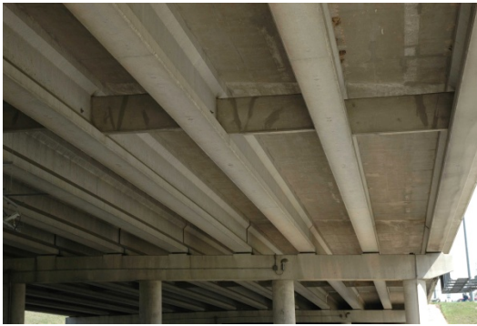
(a) Concrete Diaphragm
