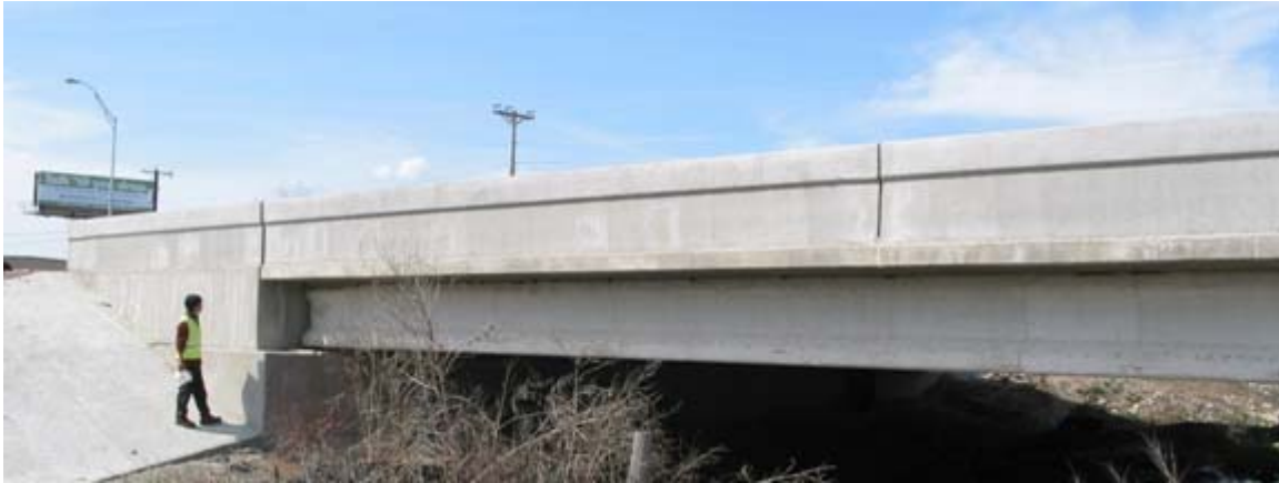
Figure 4.13 Hutto Concrete Bridge
