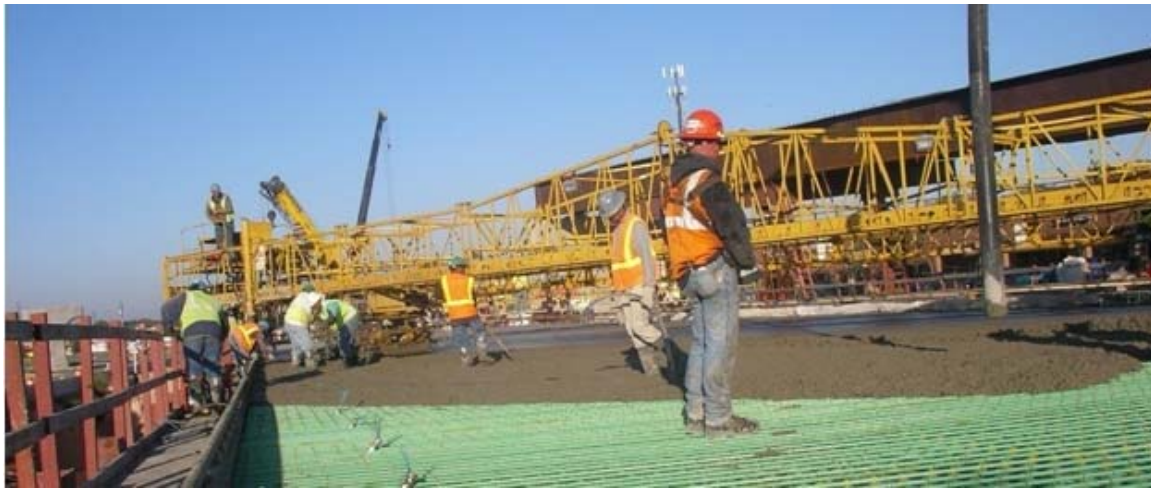
Figure 2.4 Bridge Deck Finishing Screed in Operation
