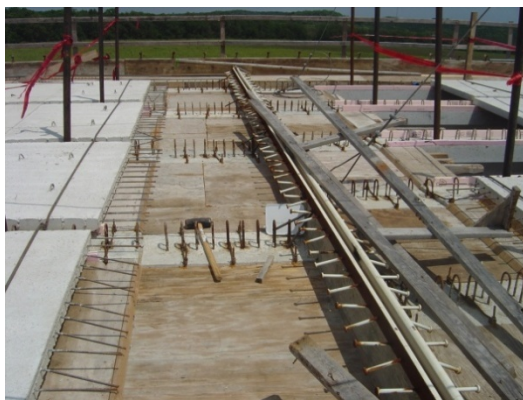
(a) Formwork for Thickened Ends
