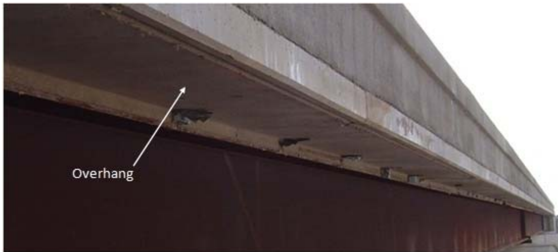
Figure 2.1 Bridge Deck Overhang
