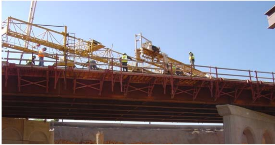
Figure 4.17 Lubbock Steel Plate Girder Bridge under Construction
