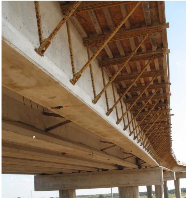
Figure 4.6 Overhang Brackets in Place
