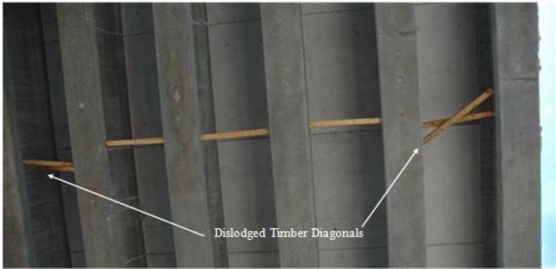
Figure 2.8 Effect of Twist on Timber Blocking
