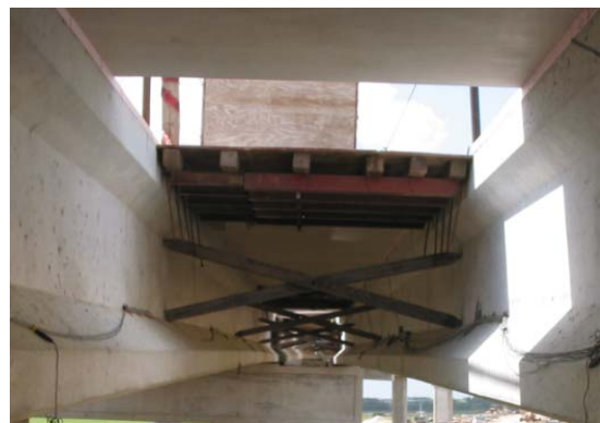
(b) Formwork Blockout for Drainage Plumbing
