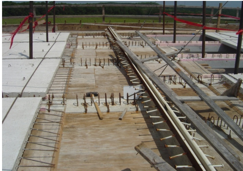
Figure 5.4 Thickened Ends in Concrete Deck at Bent Before Deck Pouring
