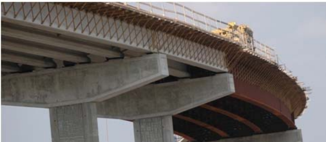
Figure 2.2 Overhang Brackets
