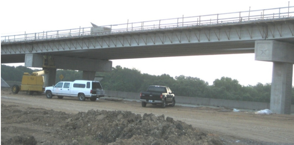
Figure 4.8 Field Measurement Span of the Airport Concrete Bridge
