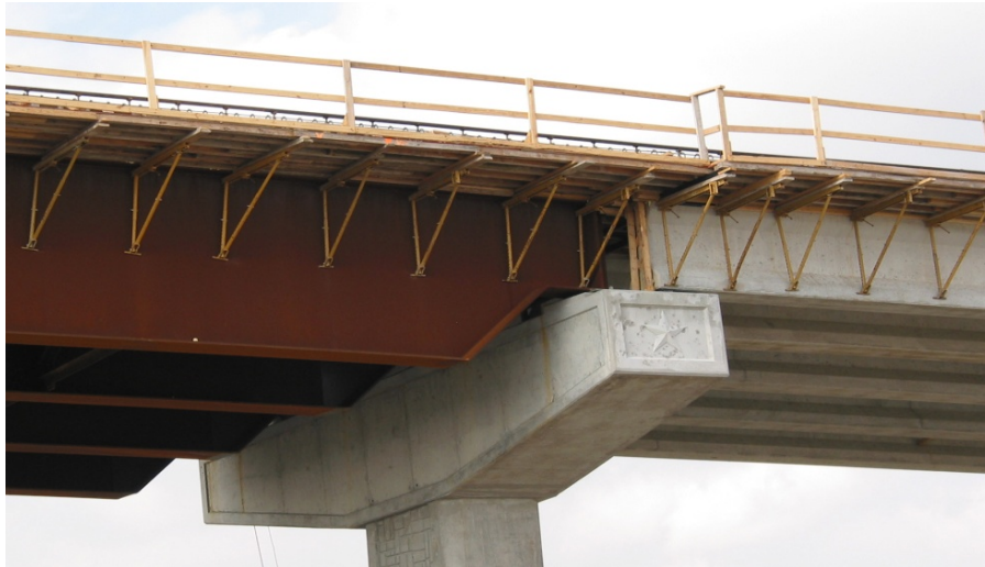
Figure 8.1 Overhang Brackets Reacting at Mid-Depth of Web
