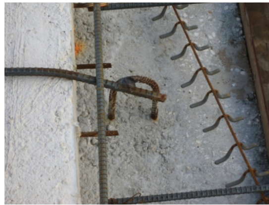
(b) Connection in Exterior Girder
