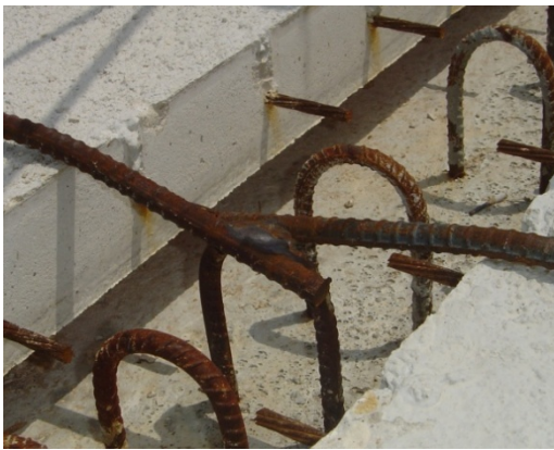
(a) Connection in Interior Girder
